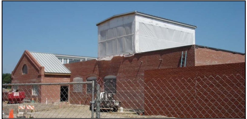
Progress on South Section of Jay Hoffman Center at Nelson
