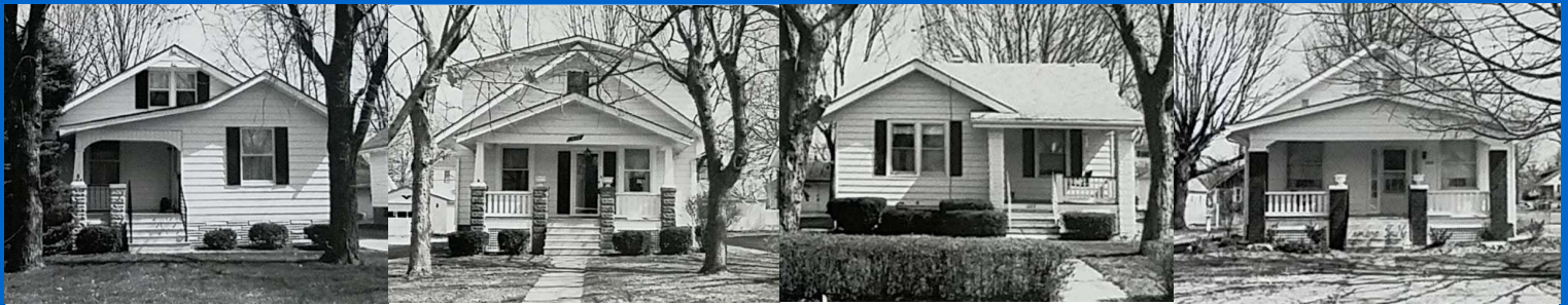
These photographs of the houses on the 1000 block of Longfellow Avenue were taken for an Edwardsville housing survey in 1995. The photographer was Steve Hughes, and the photos included his grandmother's house at 1018. The houses are, from left (North) 1018, 1020, 1022 and 1024 Longfellow Avenue. (City of Edwardsville)
