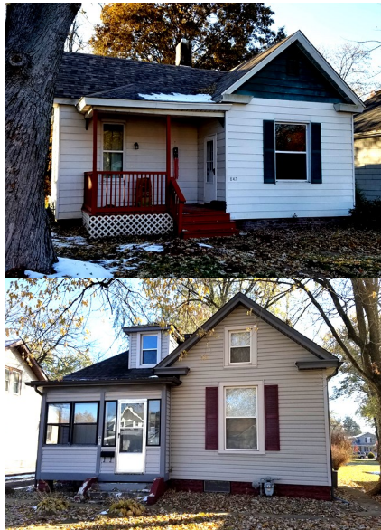
The two houses above were built for the Reid brothers. The house above, at 847 Hale Avenue was built for William Reid and the house below for John M. Reid at 828 Troy Road. Both houses likely had Victorian porches and gingerbread trim that has been lost over the years.
