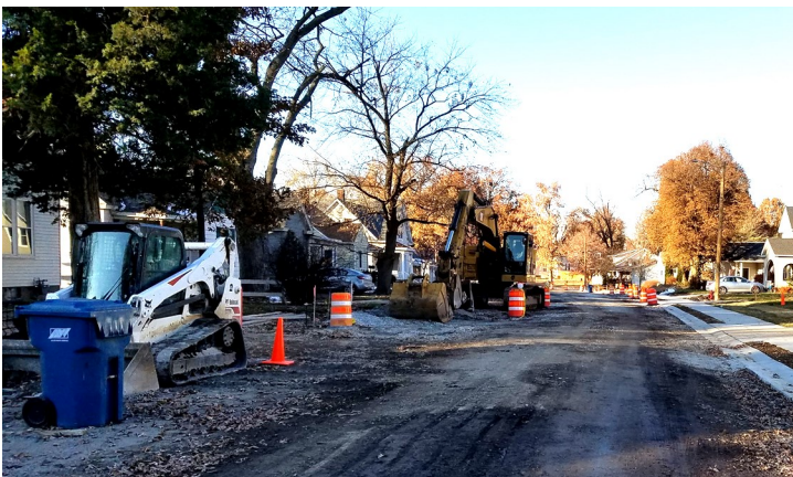
Hale Avenue construction in mid-November. (Reinhardt)
